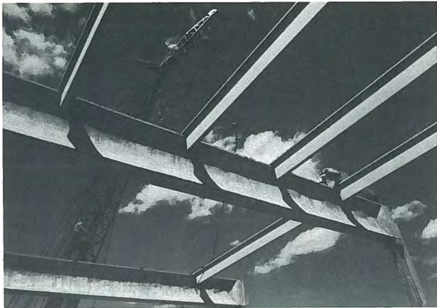
Fig. 18. Purlins framing into curved prestressed beams which used Cazaly hanger type connections. This framing system was used for many warehouses.
