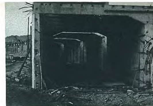
Fig. 30. Covered viaduct under construction, Rouen, France.
