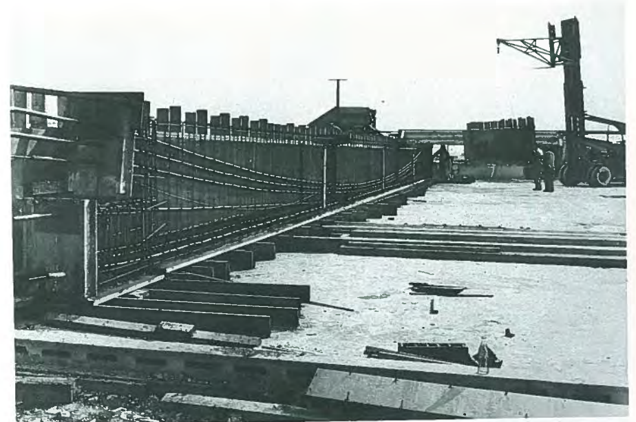
Fig. 76. Formwork for Klickitat County bridge girder showing rubber extractable cores and reinforcing in place prior to casting. Note dividers to separate beam into three segments.
