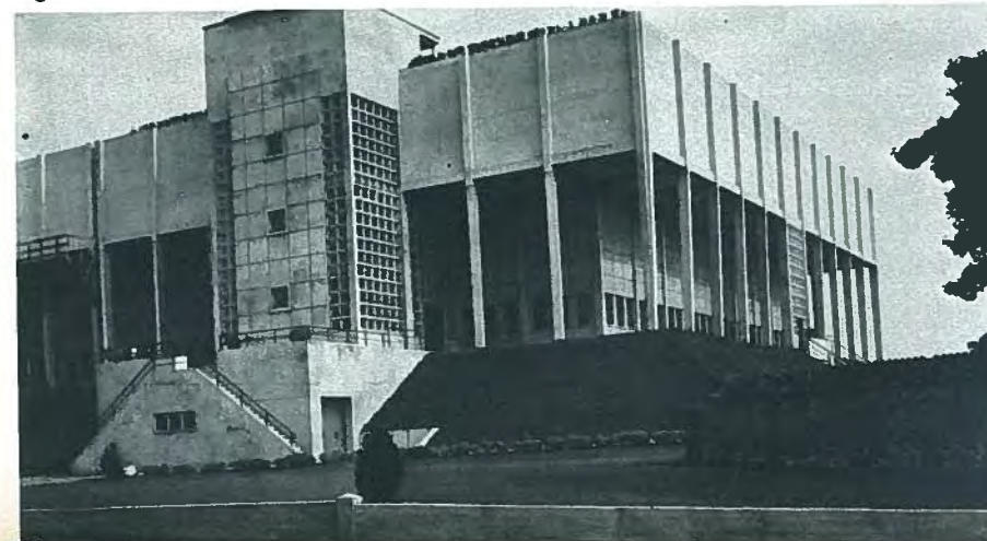
Fig. 31. Water storage reservoir and offices, Orleans, France.
