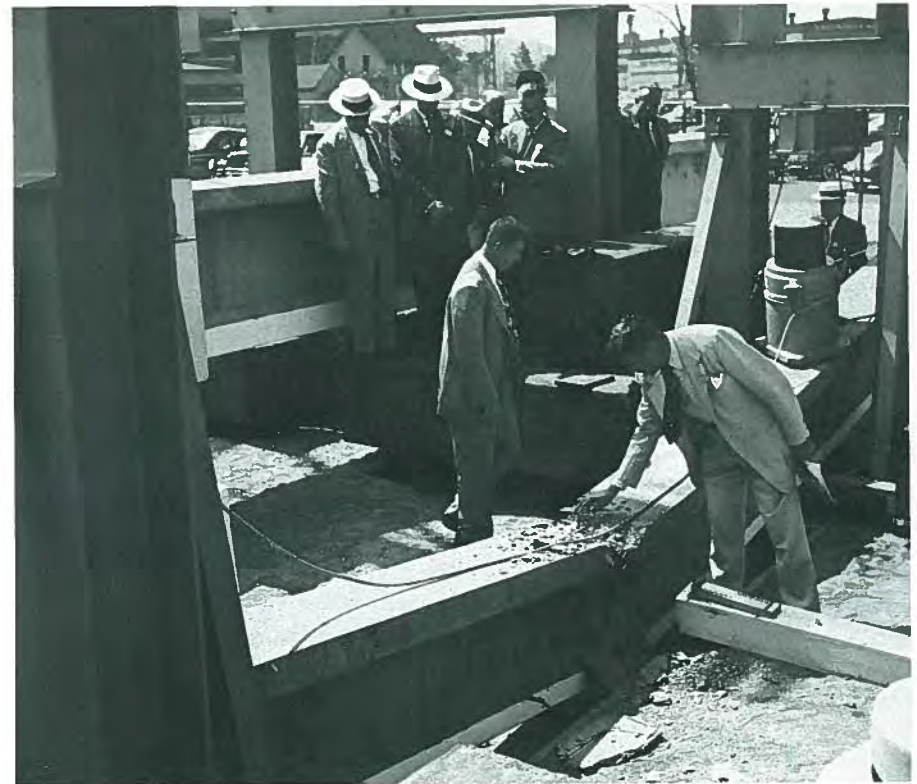
Fig. 41. After the dust settled, the author (center) and Al Waidelich inspect the fracture zone of 40-ft (12.2 m) test girder (P-40). The sudden uncontrolled failure dramatically persuaded the author to provide fully bonded tendons in all subsequent prestressed concrete construction.
