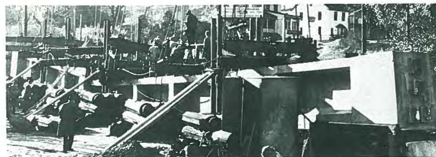
(c) Girder after failure.
