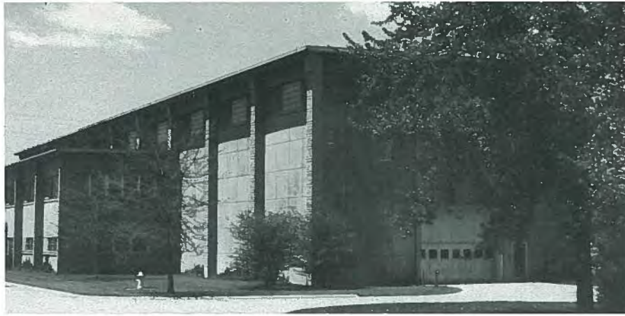
Fig. 36. PCA's fire test center.
