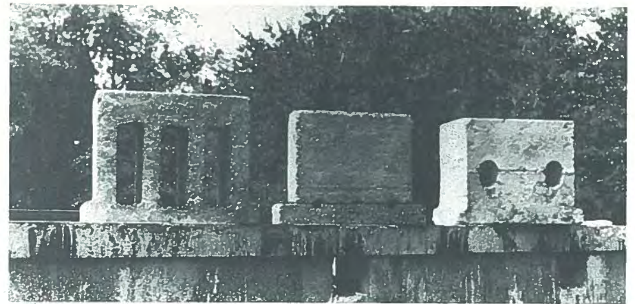
Fig. 4. Madison County Bridge beam units.
