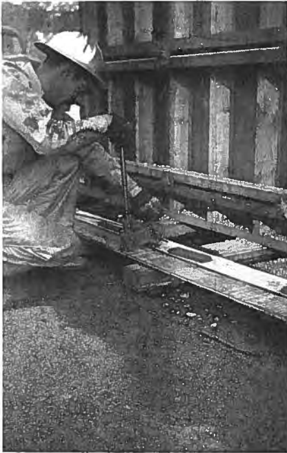
Fig. 5. Wooden trough for measuring and cutting wire.
