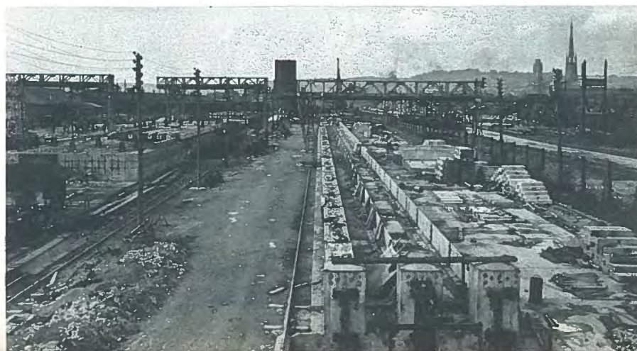
Fig. 29. Prestressing yard for segments of covered viaduct, in Rouen, France.
