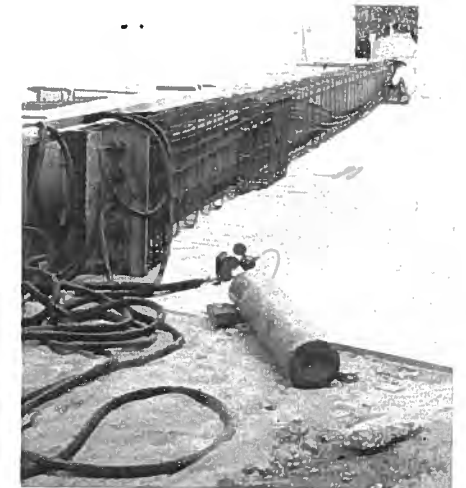
Fig. 19. Forms with inflatable rubber voids.
