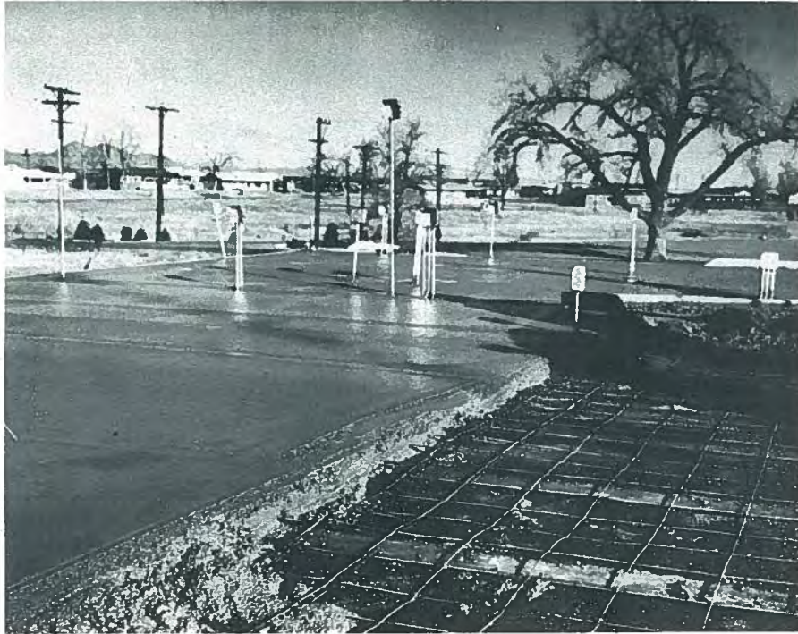
Fig. 27. In the final operation, concrete is placed and finished over the form board covering the Quadeck.
