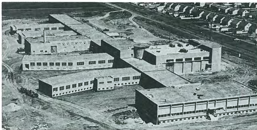
Fig. 8. School for the Deaf, Edmonton, Alberta, 1955—complete precast column and beam framing and prestressed double tee floor and roof slabs.
