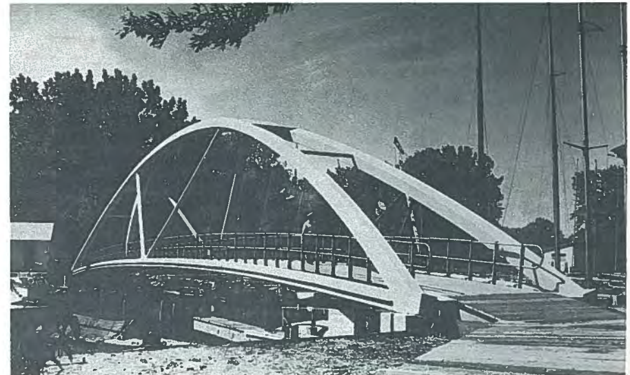
Fig. 14. Prestressed concrete footbridge for the Royal Canadian Yacht Club of Toronto, designed by L. G. Cazaly.
