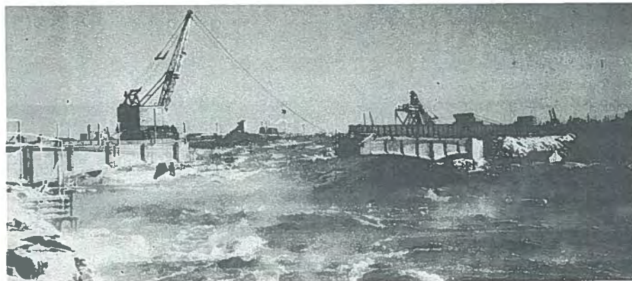
Fig. 19. The three-span Nelson River Bridge under construction in Manitoba (1957).
