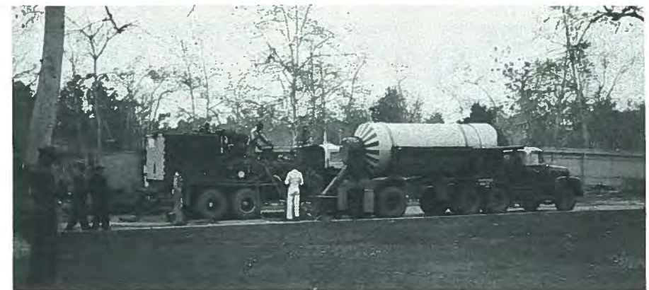
Fig. 11. Halliburton grouting the girders.
