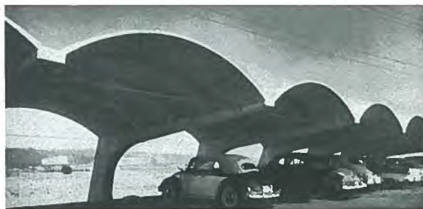
Fig. 51. Precast prestressed concrete barrel shell carport for Concrete Engineering Company (1953).
