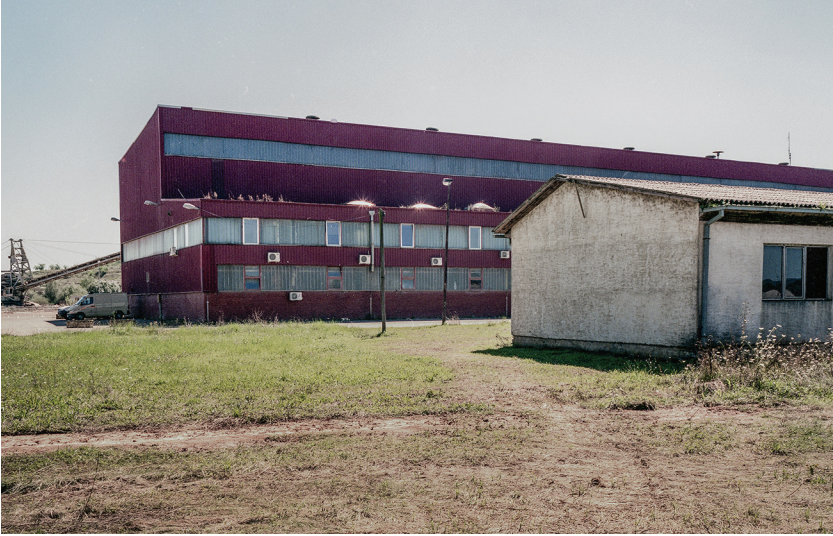
Figure 8. The main building and the infamous white house at Omarska mine near Prijedor, used as a camp in 1992. (Courtesy of Pawel Starzec.)
