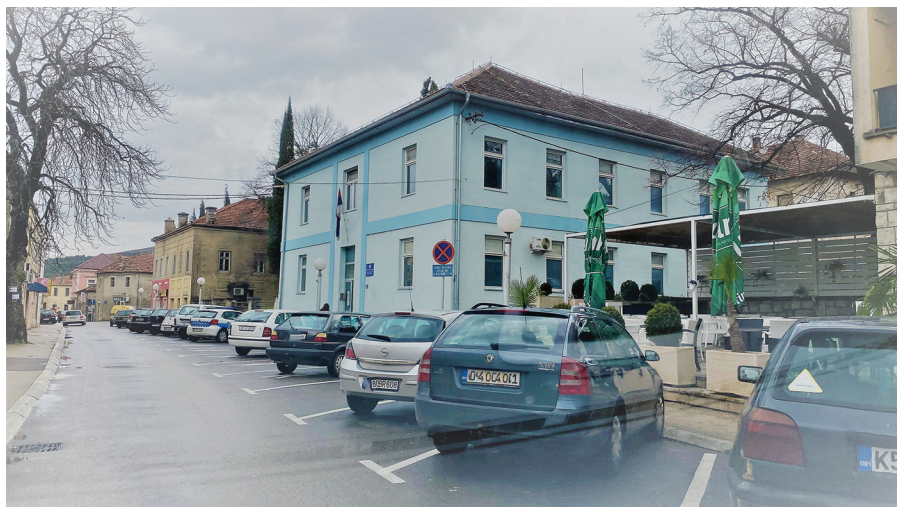
Figure 14. The police station in Bileća, used as a detention facility for Bosniak civilians in 1992. (Courtesy of Sadmir Mustafić.)
