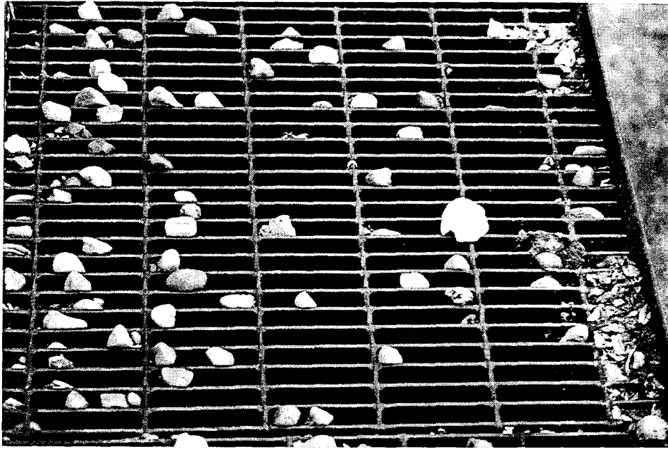
Figure 9. Blinded-off bar grate separation screens
