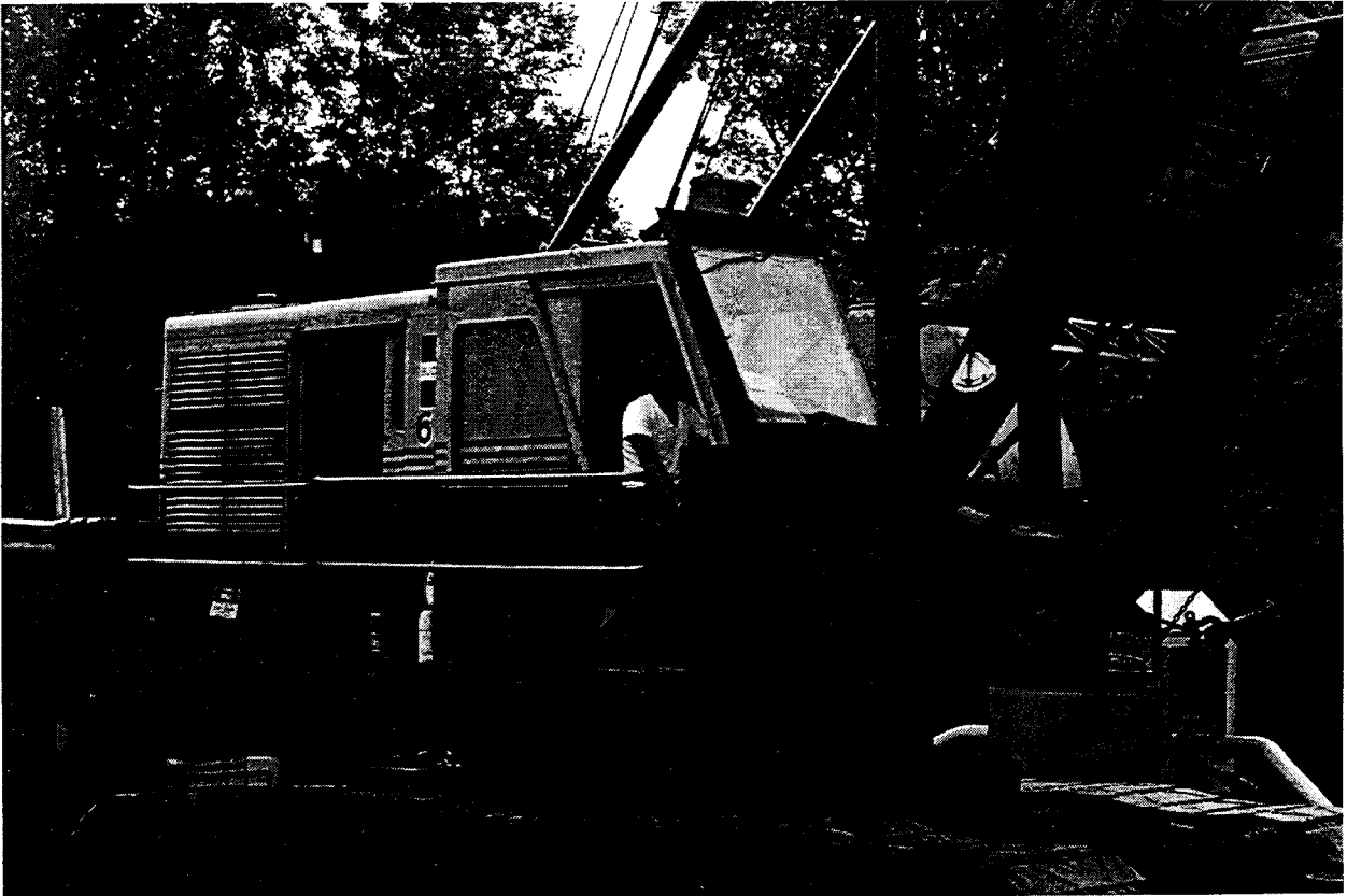
Figure 2. Crane operator's protective barrier
