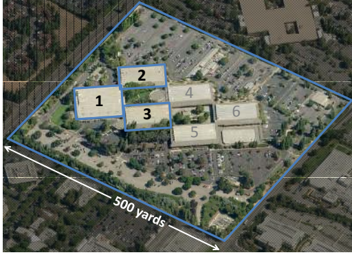
Figure 1. Aerial view of the campus, showing the six main buildings, three of which are currently instrumented for power monitoring.
