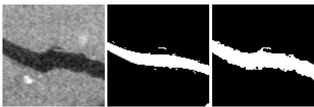
Figure 8: Section from NC12 with a curved crack structure and thin branching (left). Sections after applying the Frangi filter with hysteresis binarization (middle) and HP (right).
