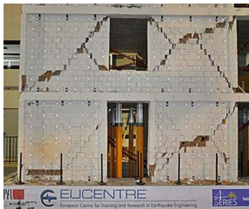
Fig. 12.16 URM walls of shake table test unit after Run 9 (Beyer et al. 2014)
