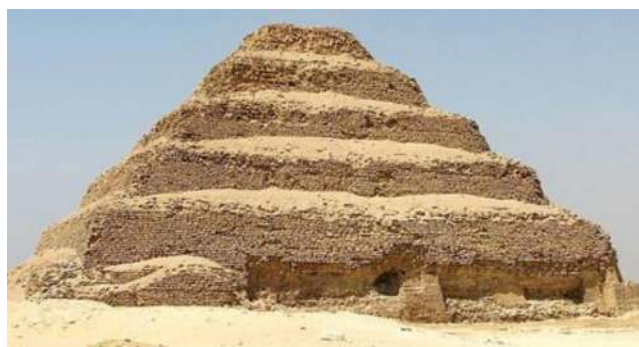
FIG. 8. The tomb of Pharaoh Djoser (actual name, Netjerykhet, second King of the Third Dynasty, Old Kingdom; ruled from ~2667 to 2648 BC). 22 This is the first pyramid constructed of cut stone (uncut-stone pyramids in Caral, Peru, are of a similar age). 26 The Djoser Pyramid was initially 62 m tall, with a base of 109 \times 125 m 2 , and clad in smoothed white limestone. 24 Sometimes called the Step Pyramid, it consists of six mastabas (rectangular structures with sloping sides), the first of which is square. Photograph attributed to Roweromaniak, Poland, licensed under Creative Commons Attribution-Share Alike 2.5.
