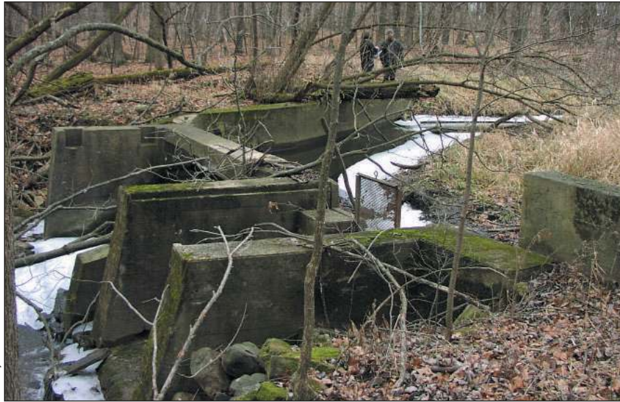
Figure 1. The Boulder Creek dam, Wisconsin was constructed during the 1930s as part of a fish hatchery operation. The impoundment is now completely filled with sediments and has been colonized by grasses and weeds. The structurally compromised dam is scheduled for removal in 2003.
