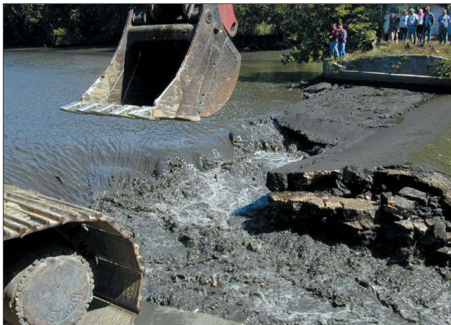
Figure 2. A torrent of muddy brown water is released following the breaching of the Rockdale Dam, Wisconsin. Downstream concentrations of suspended sediment increased by three orders of magnitude over a 2-hour period and remained elevated over the next 3 days.
