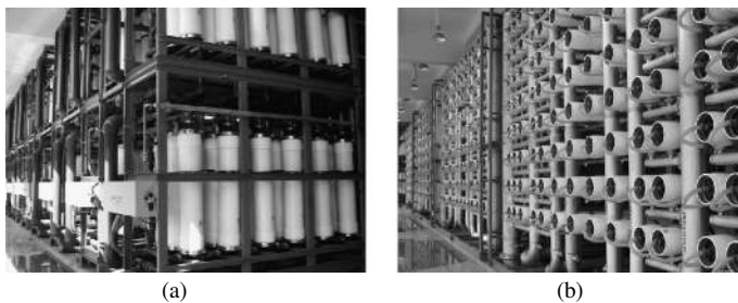
Figure 4.6 Full-scale integrated membrane system (IMS) of Caotan water purification plant for tap water supply located at Kaohsiung County, Taiwan (a) Ultrafiltration system; (b) NF-LPRO system. The total land area of IMS is 1380 m 2 . (Photos provided by KINTECH Technology Co., Ltd.)
