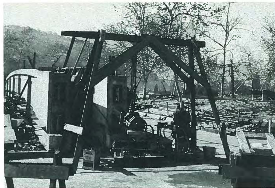
Fig. 10. Stressing the Arroyo Seco girders.
