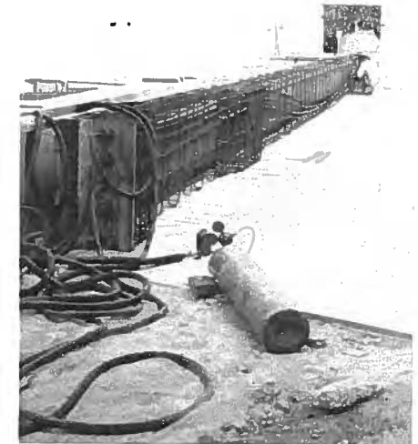
Fig. 19. Forms with inflatable rubber voids.
