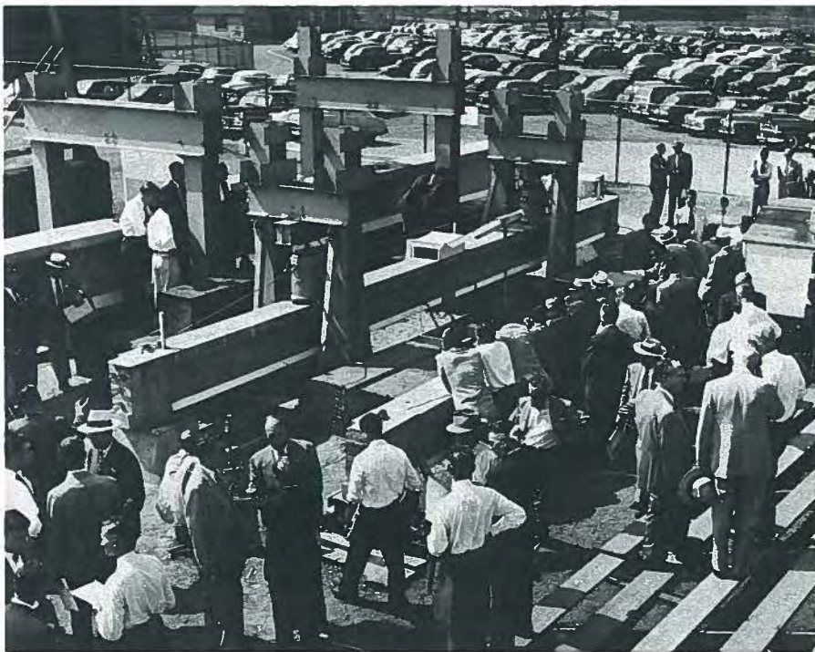
Fig. 37. An overflow crowd of invited guests witnessed the Austin Company tests in 1951. Three full-scale girders [two 40-ft (12.2 m) and one 60-ft (18.3) girders] were load tested using hydraulic jacks.
