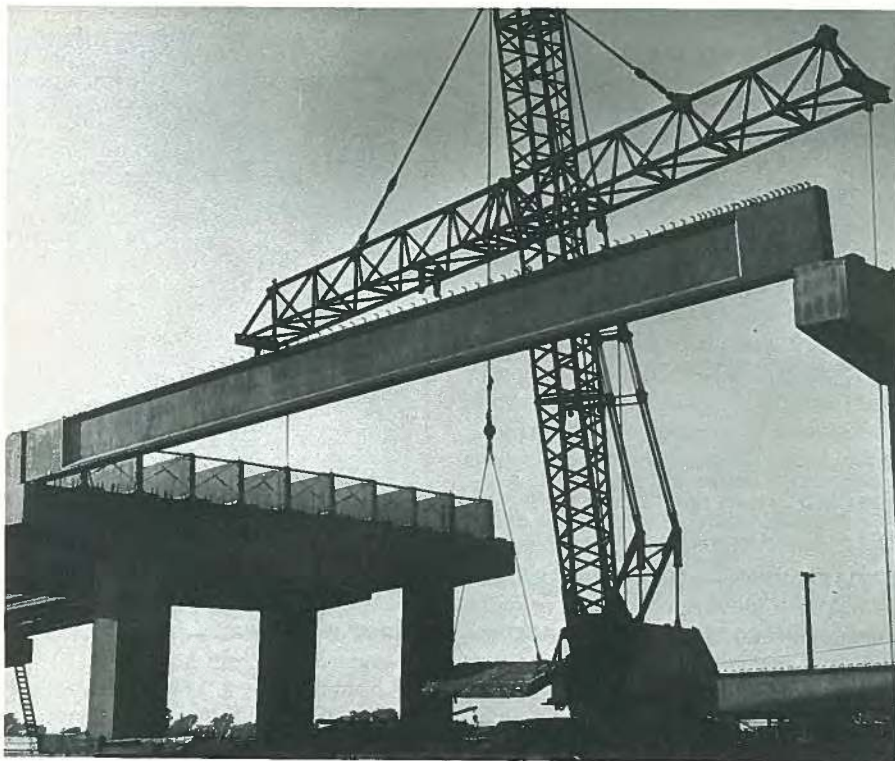
Fig. 49. Napa River Bridge, 1957: one of the earliest applications of pretensioned deflected strands. Design by California State Department of Highways.
