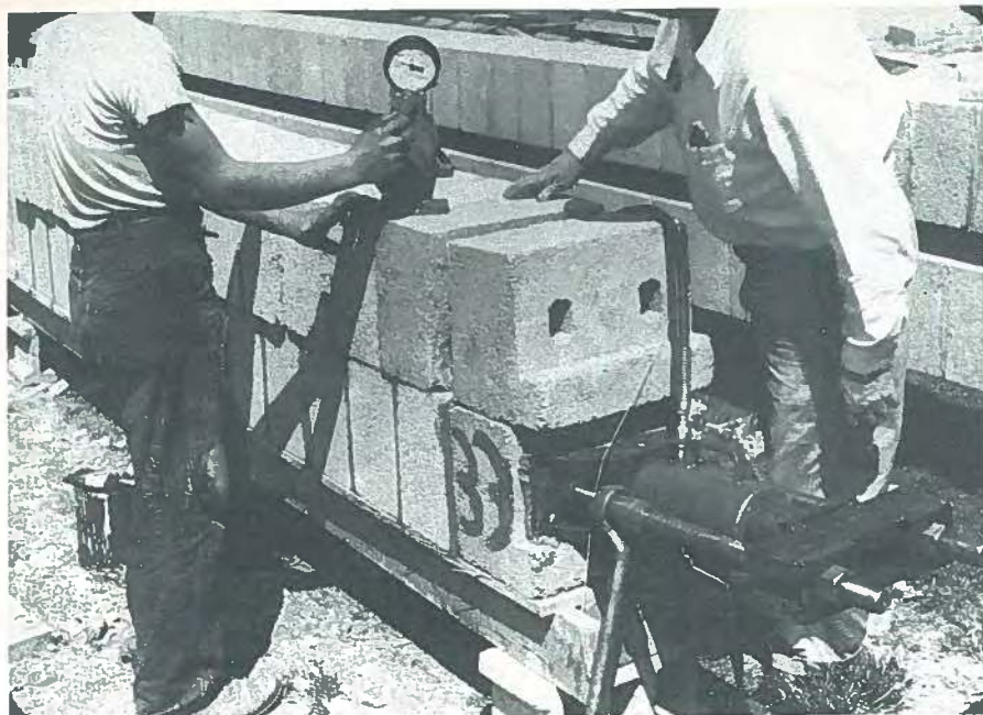
Fig. 2. Tensioning stadium beams.
