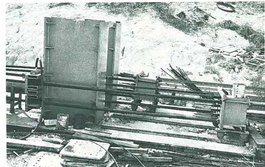
Fig. 33. Early multi-strand tensioning of an 18-in. (457 mm) square pile. Courtesy: Dura-Stress, Inc., Leesburg, Florida.
