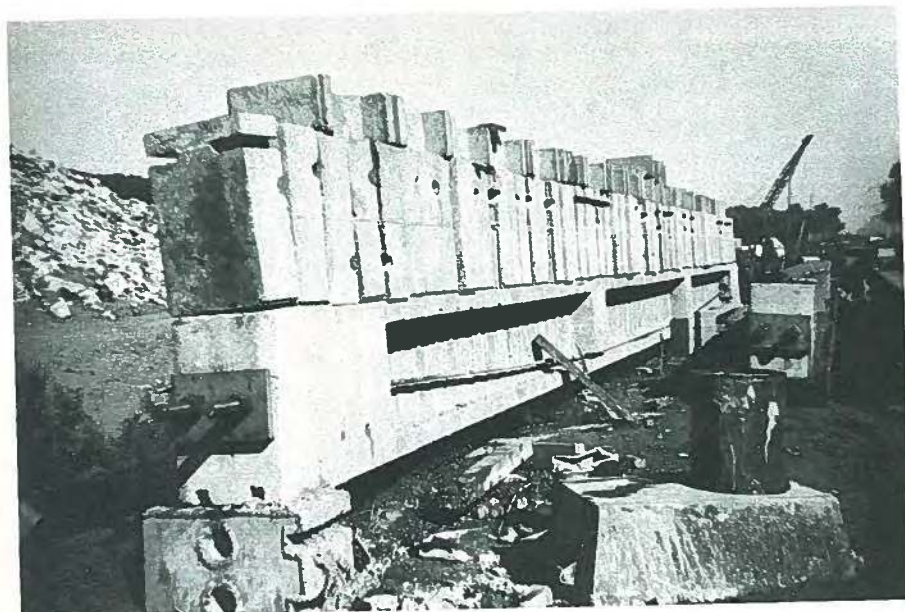
Fig. 15. Testing of Michigan block-beam with 1.5 live load.
