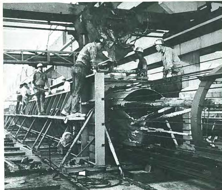
Fig. 83. Formwork and reinforcing cage for casting pretensioned cylinder piles.
