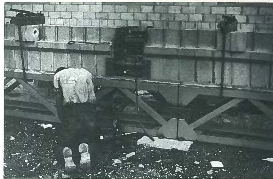
Fig. 10. Tensioning two 16x24-in. (406 x 610 mm) block building beams by jacking them apart.
