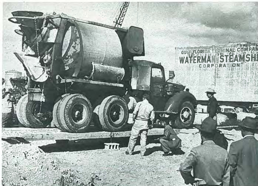
Fig. 24. Demonstration test by Cone Brothers Construction Co. in Tampa, Florida (1954) of 2-in. (51 mm) thick prestressed slab with 4-in. (102 mm) composite topping. The span was 30 ft (9.2 m) long.
