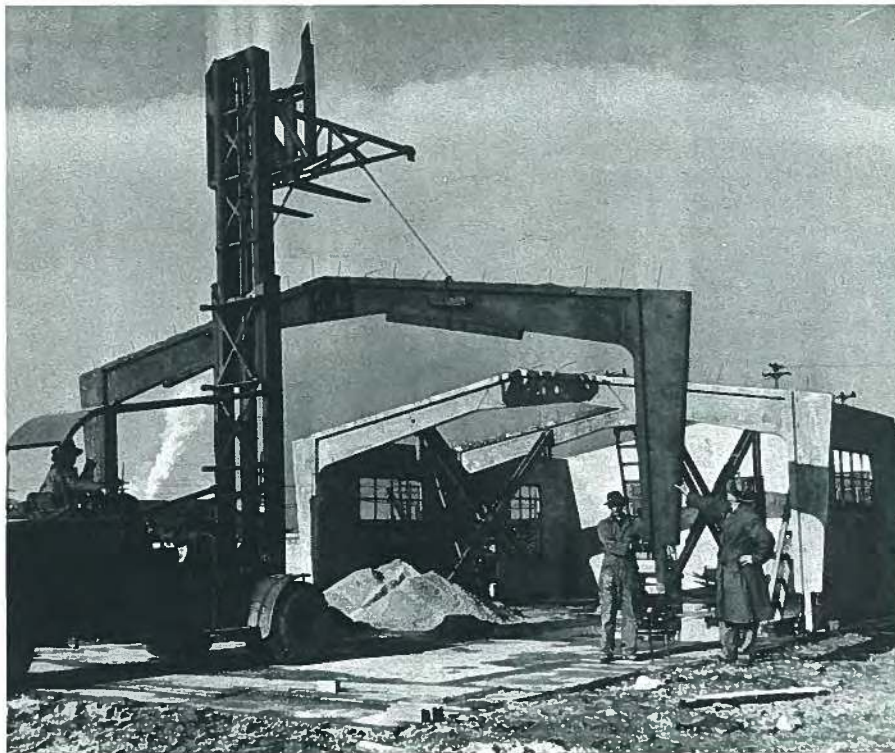
Fig. 43. Erection of Concrete Engineering Company shop building (1951).
