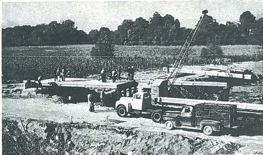
Fig. 10a. Erection of block-beams hauled 176 miles from fabricating plant to erection site, Obion County, Tennessee (about 1950).
