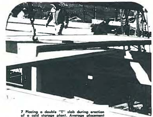
7 Placing a double "T" slab during erection of a cold storage plant. Average placement time was three minutes per slab.
