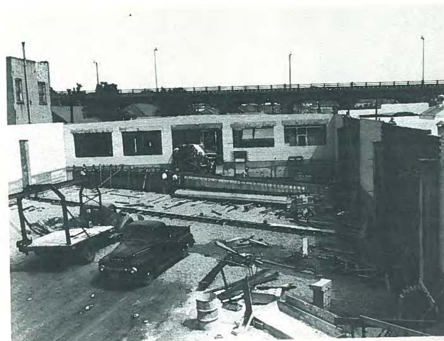
Fig. 22. Post-tensioned beams were cast on site at the Star Bakery because of the limitations of existing transportation equipment.
