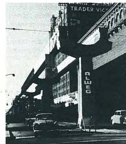
Fig. 88 View of the Seattle Monorail under construction, showing the cross section of the girders, and the shape of the support columns, on a straight stretch of the beamway.
