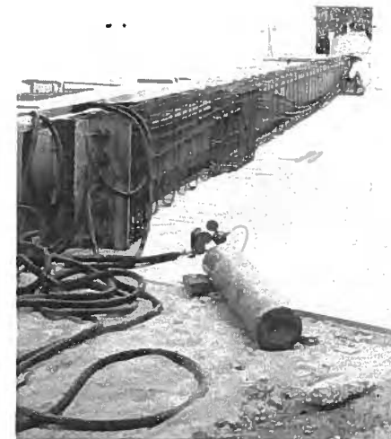
Fig. 19. Forms with inflatable rubber voids.
