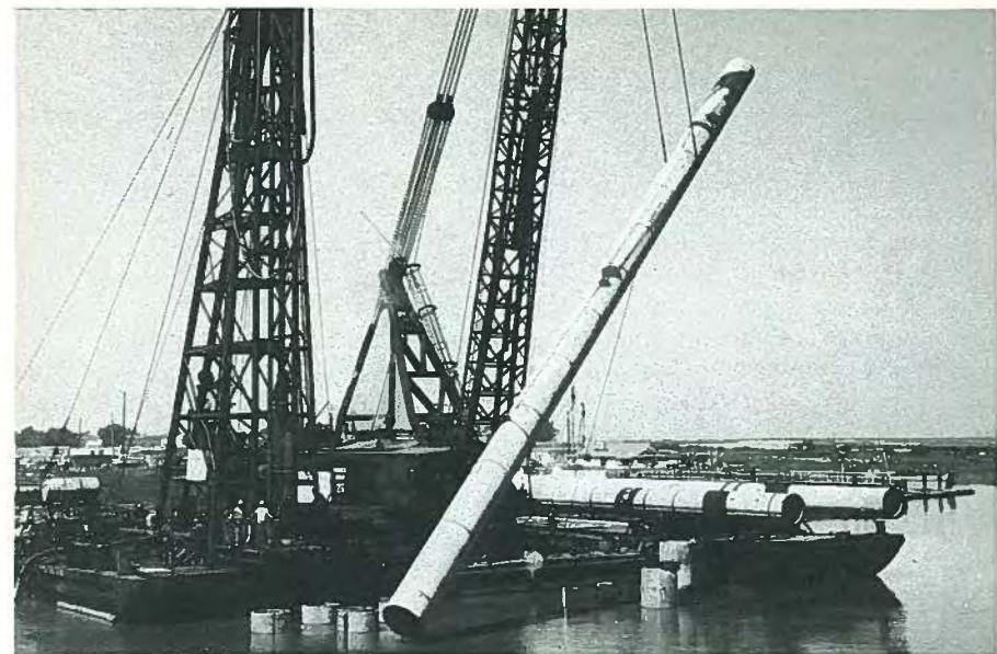
Fig. 52. Napa River Bridge, California: pretensioned monolithic cylindrical pile, 54 in. diameter, 120 ft long. It is believed to be the first such pile used worldwide.
