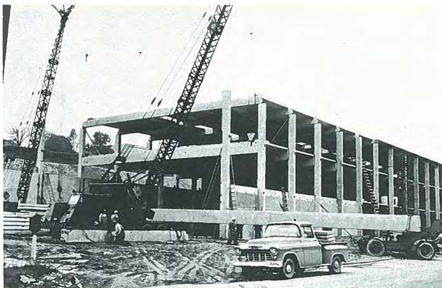
Fig. 66. Erection proceeds on totally precast three-story school in Tacoma.
