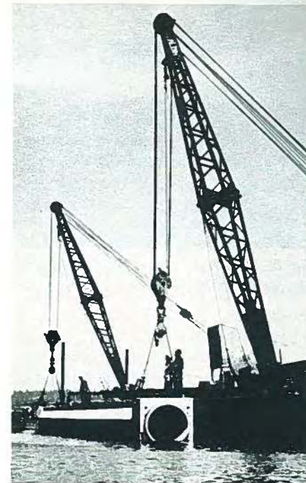
Fig. 87. 85-ton (77 t) precast prestressed hollow pipe section being installed in Lake Washington.
