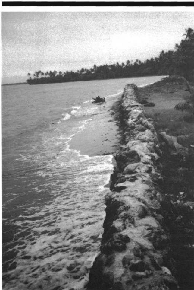
Plate 3. Seawall in front of Nukui village.
