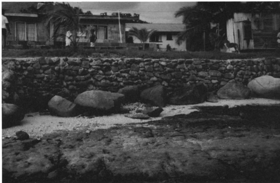
Plate 9. Vertical seawall with toe protection by large stones.
