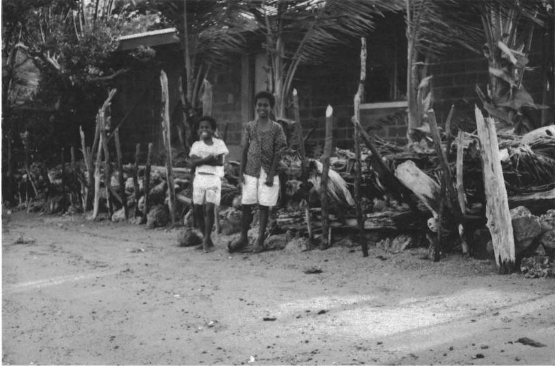
Plate 5. Traditional coastal protection by wooden poles poked into the sand with sand and rubbish piled behind them.
