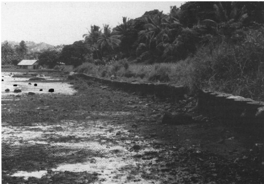
Plate 8. Vertical seawall of drums with concrete inside.
