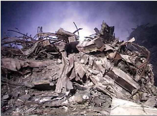
Figure 4. View of the rubble near WTC Tower 2 and Building 4 showing pancaking and the lack of voids.
