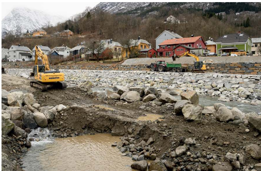
FIG. 3. During a visit to Odda in Mar 2017, some of the Hordaklim researchers got to see the extensive repairs being done to the River Opo after the flooding episode in Oct 2014 (Pontoppidan et al. 2017). Photo by Erik Kolstad.
