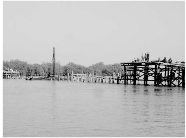
Fig. 7. Destruction of wooden bridge to Plautonton Island.
