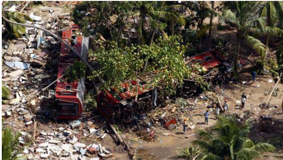
Figure 11. Overturned rail carriages near Peraliya on the south-west coast.
