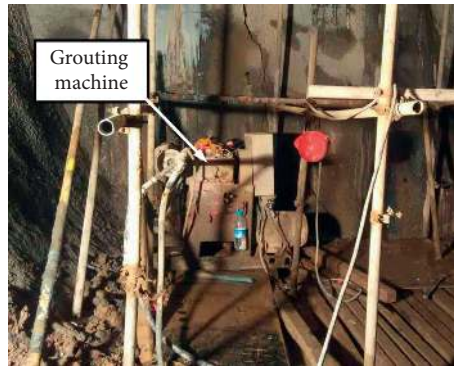
FIGURE 7: In situ grouting equipment and environment.
