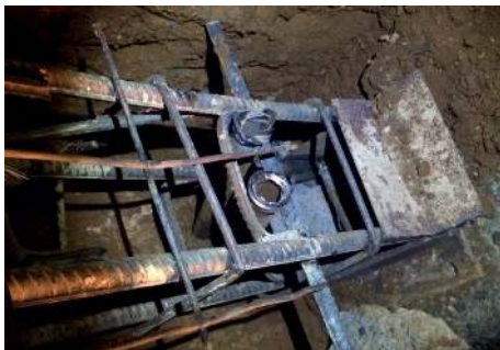
FIGURE 13: Connection of lock pin anchor pipe on-site.
