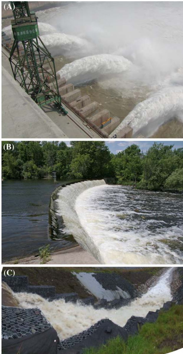
Fig. 1 Air entrainment in hydraulic structures (a) Free-surface aeration at the bottom outlet of the Three Gorges Dam, China on 20 October 2004— Q_w = 1700 \text{ m}^3/\text{s} per jet, V_1 = 35 \text{ m/s} , d_1 = 7 \text{ m} , W = 9 \text{ m} (b) Plunging jet aeration at the toe of Nicholson's Dam, Canada in June 2006 (Courtesy of Ken WATSON) (c) Interfacial aeration down a stepped chute on 8 June 2007 (Courtesy of Tony MARSZALEK)—Stepped chute: \theta = 18.4^\circ , h = 1 \text{ m} , l = 3 \text{ m} , W = 8 \text{ m} , flow from top left to bottom right
