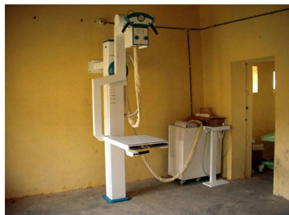
Figure 2 Nyaya Health X-Ray Installation. Note the protective screen around the control room had yet to be installed in this photograph.
