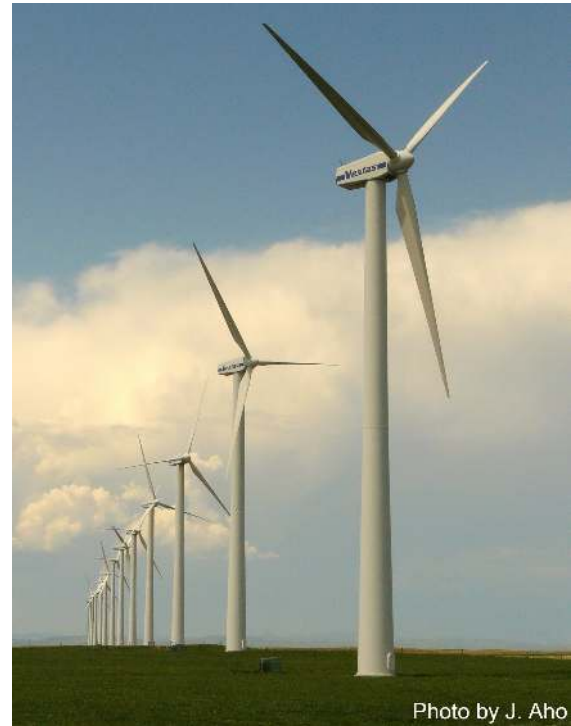
Fig. 1. A row of turbines in a wind plant located in Alberta, CA. This wind plant contains 114 horizontal axis wind turbines (HAWTs), each rated at 660 kW with a rotor diameter of 47m and hub height approx. 50m.
