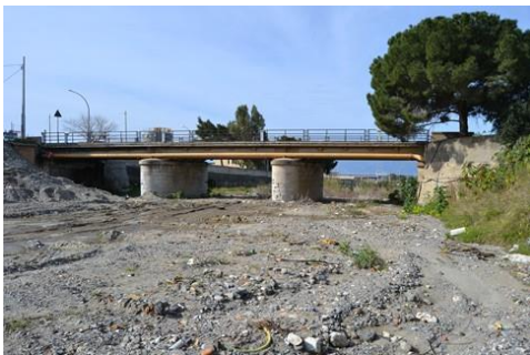
Figure 2. Detail of the San Gregorio Bridge
