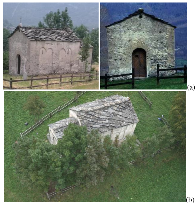
Figure 2.(a) Two detailed view of the S. Maria's Chapel; in (b) it is visible how a part of the object is hidden by trees, which can be a problem for the use of the oblique images to build a part of the complete 3D model
