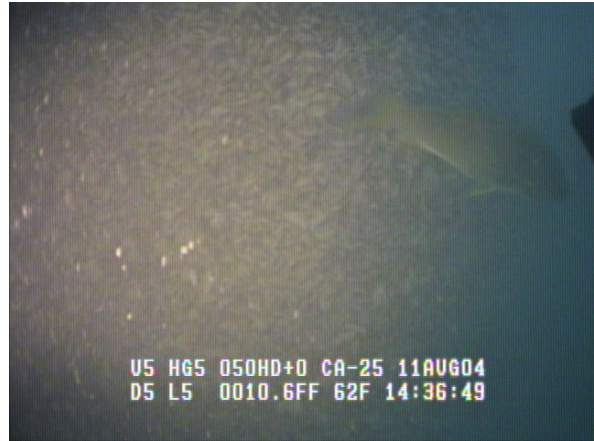
Fig 11: A seawall inspected in Calumet harbor
