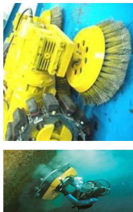
Figure 5. Brush based underwater surface cleaning
