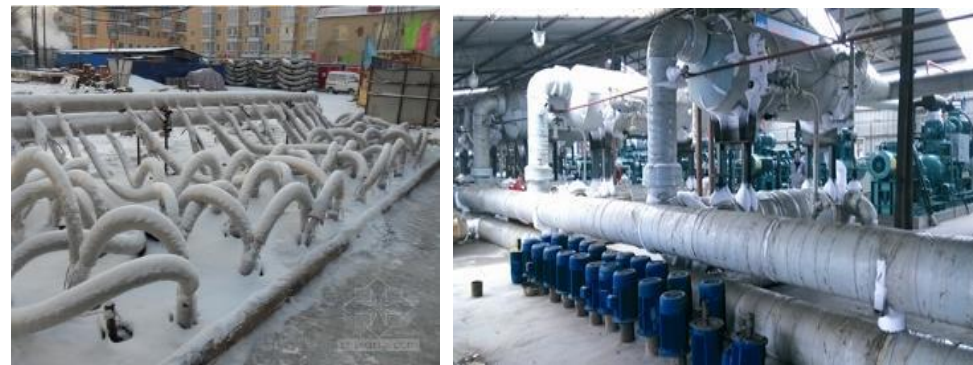
Figure 22. Artificial freezing method application [138].
