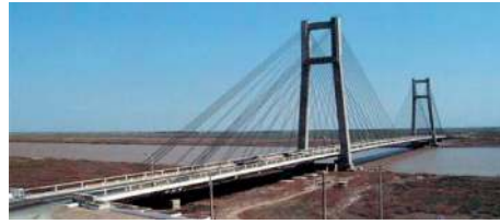
FIGURE 9: Tianjin Yonghe bridge [41].
