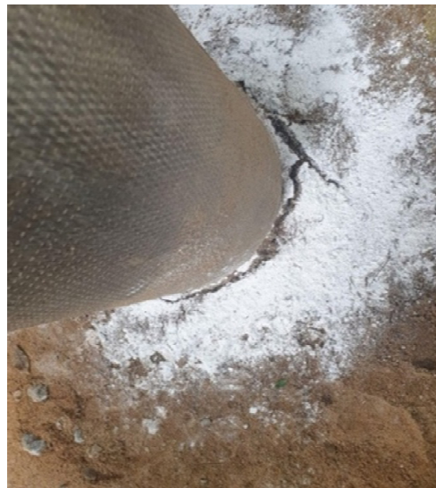
Figure 15. Gap between pile and soil.
