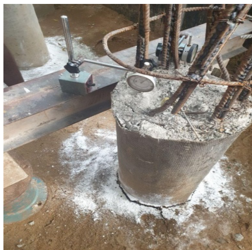
Figure 16. Deflection of the piles during the uplift.
