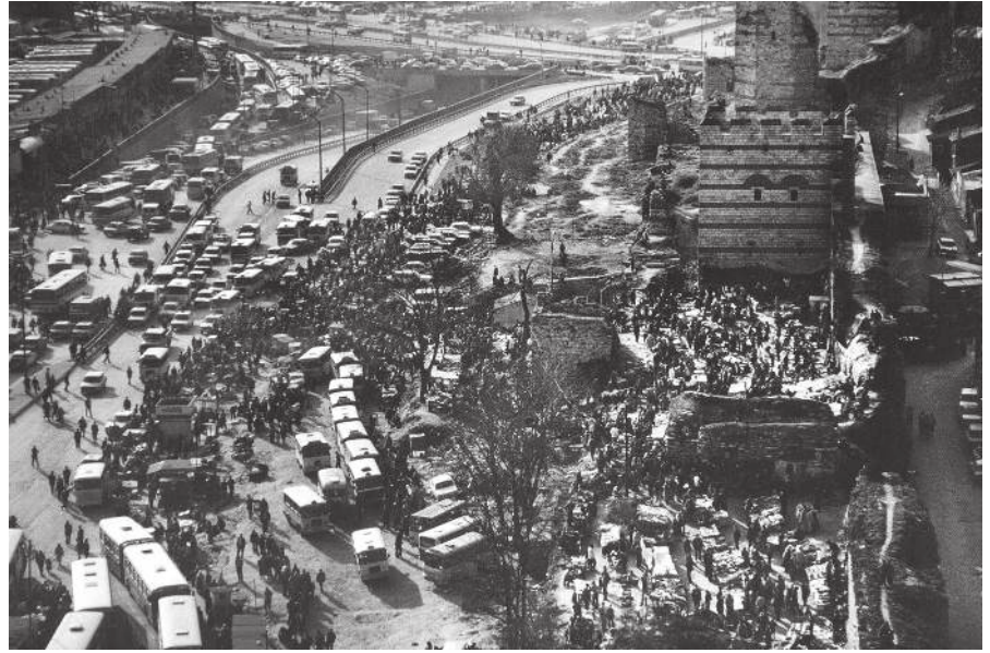
Figure 14. The Intercity Bus Terminal and Open Market Area at Topkapı (Kalfagil, 2008, 184).
