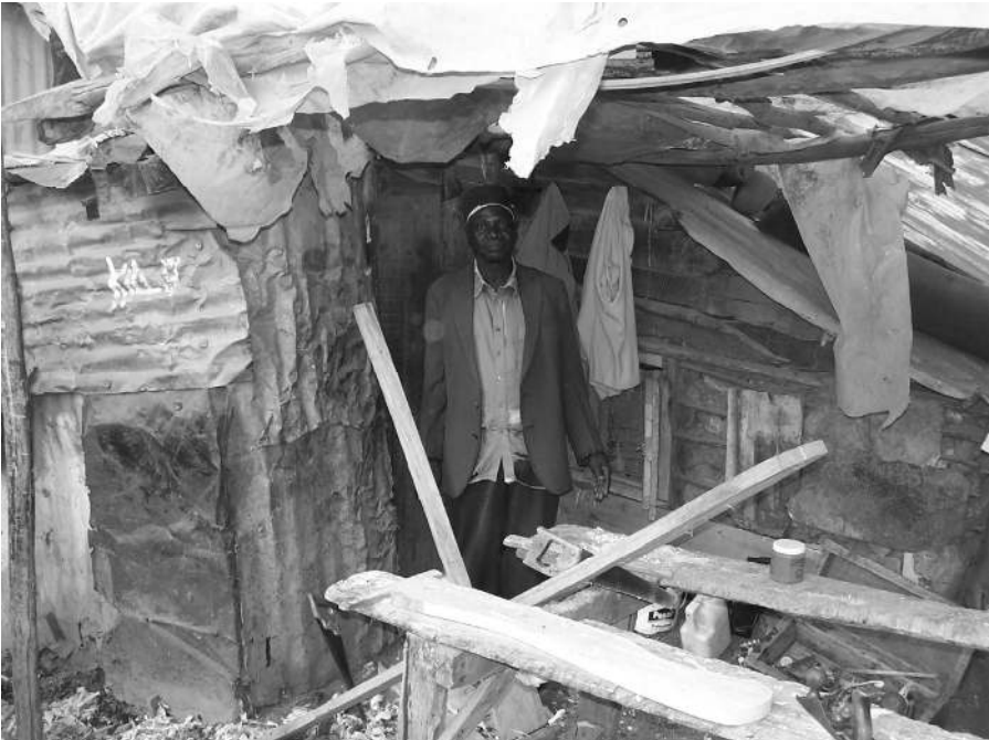
Photo 7.2: Shelter quality: GSS in Ghetto-Huruma, old iron sheets, polythene, wooden walls, mud floor
