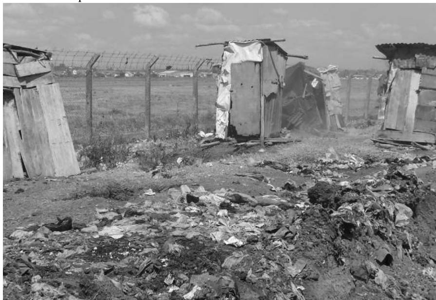
Photo 7.8: Mitumba: private old iron sheet, wood, polythene latrines, right next to Wilson Airport
