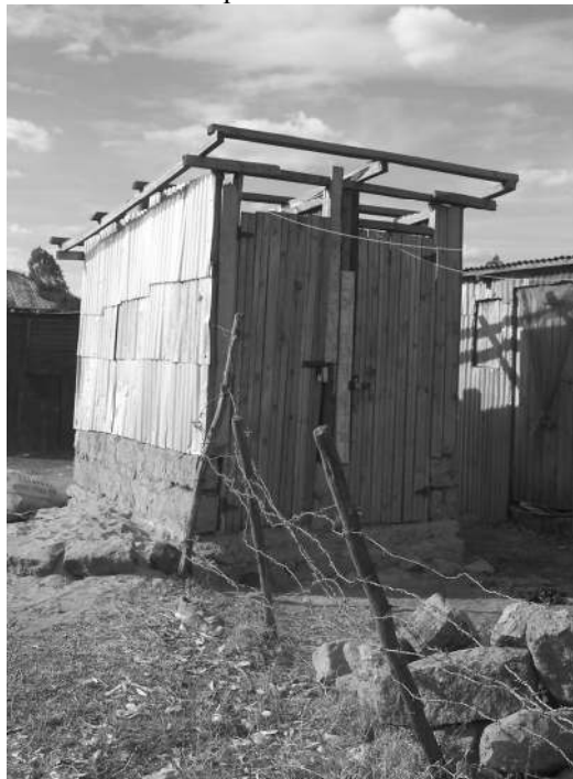
Photo 7.9: BHC: private stone/new iron sheet pit latrine
