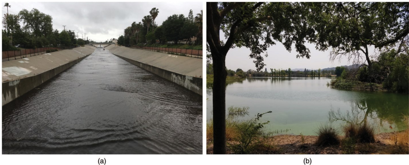
Fig. 5. (Color) (a) Historically, urban stormwater has been managed for flood control with large pipes, concrete channels, and aqueducts, such as the Los Angeles River; (b) Increasingly, stormwater is viewed as a resource, and may provide water for beneficial uses as well as ecosystem services, for example, the Los Alamitos Percolation Ponds in San Jose (Images by authors.)
