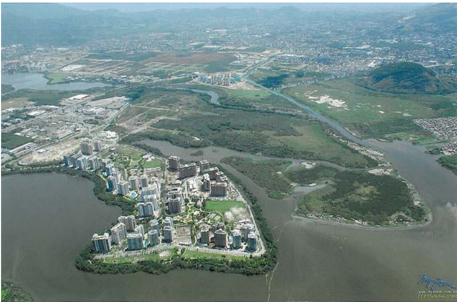
Fig. 29.6 Aerial view of the Peninsula and Gleba F in 2012, after development and establishment of the three parks: two along the lagoon in the left side, and the large green area on the right side. (Photo taken by and published with kind permission of © Carvalho Hosken S.A. 2012. All Rights Reserved)
