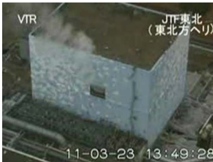
Figure 16. 1F2 reactor building with open blowout panel. (Courtesy of TEPCO [119])
