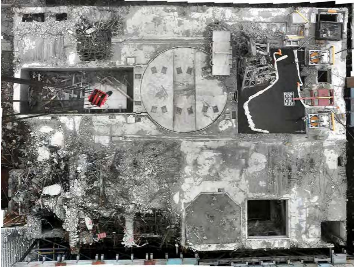
Figure 33. Damaged areas on 1F3 reactor building floor plan. (Courtesy of TEPCO, [15])
