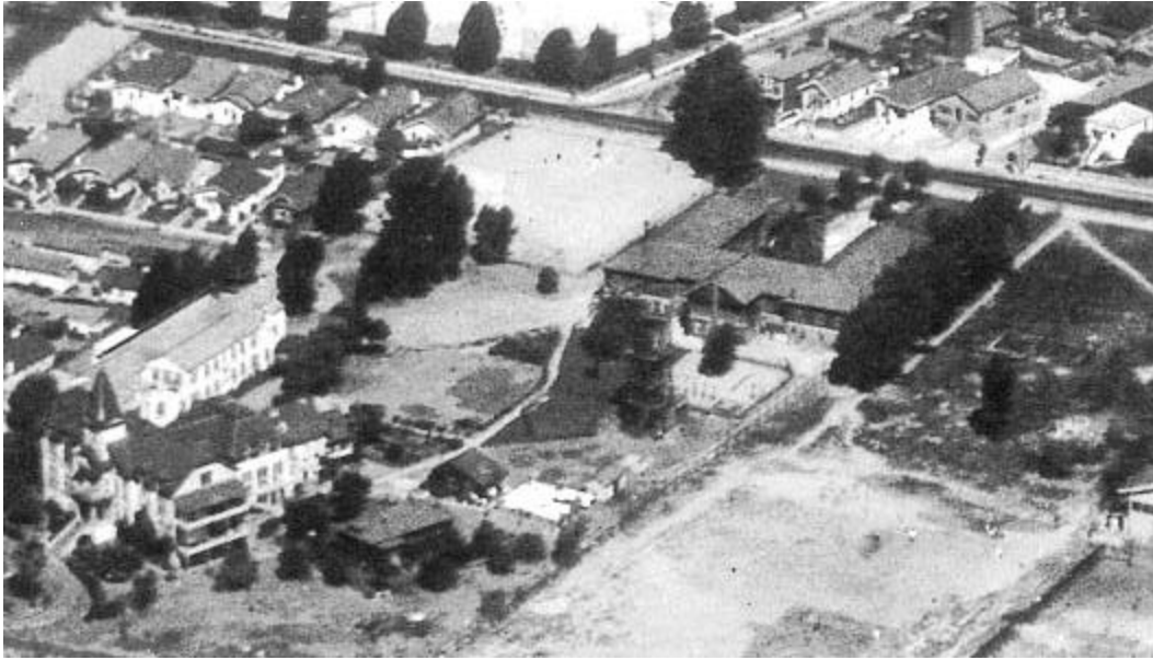
Figure 3. The Children's Home, c. 1925. The main entry of the Children's Home faced 45 th Street after it was rebuilt in 1906. The "new" Babies' Home, completed in 1925, is next to the Home for Aged Women, erected in the early 1880s. Use courtesy of The Oakland Museum of California.
