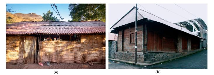
Figure 16. Substitution of the traditional roofing systems: (a) Bajareque house in Santa Cruz de Morelos; (b) Troje in Charapan.
