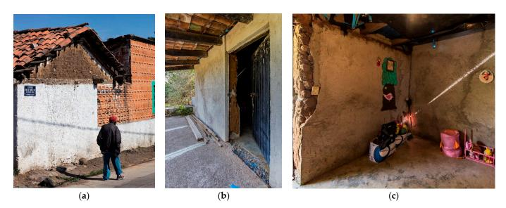
**Figure 14.** Constructive malpractices and modifications on adobe dwellings: (**a**) Invasion of the traditional wall in San Nicolás Obispo; (**b**) Cement coating in Tacícuaro; (**c**) Cement coating and pavement in Tacíacuaro.
