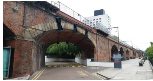
(b) Pictorial view of the bridge
