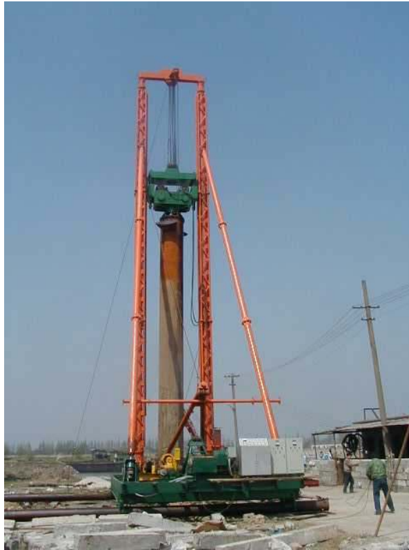
Figure 3 Picture of PCC piling machine
