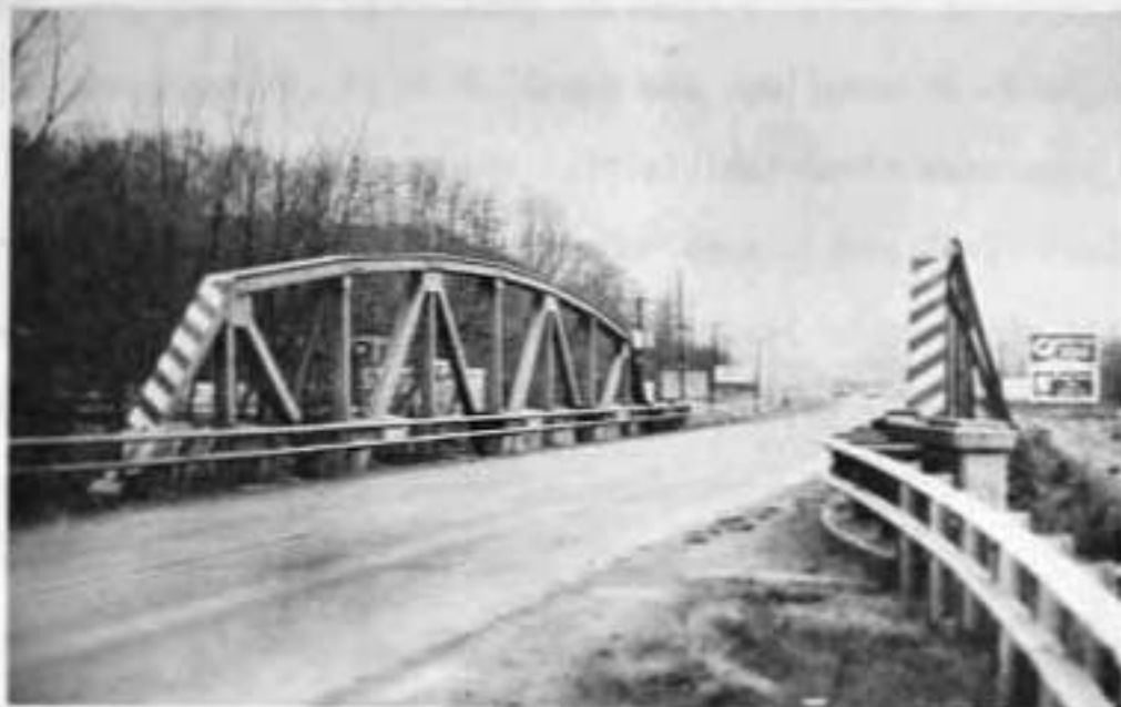
Figure #1. Bloomington Bridge SR-37
