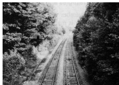
(b) Mature tree growth (Sycamore) on a cutting
