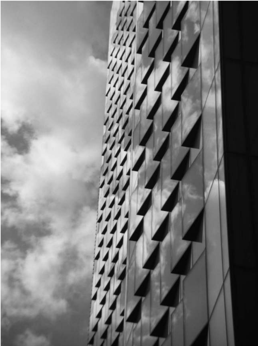
Picture 2. The façade of Ropemaker Place.
