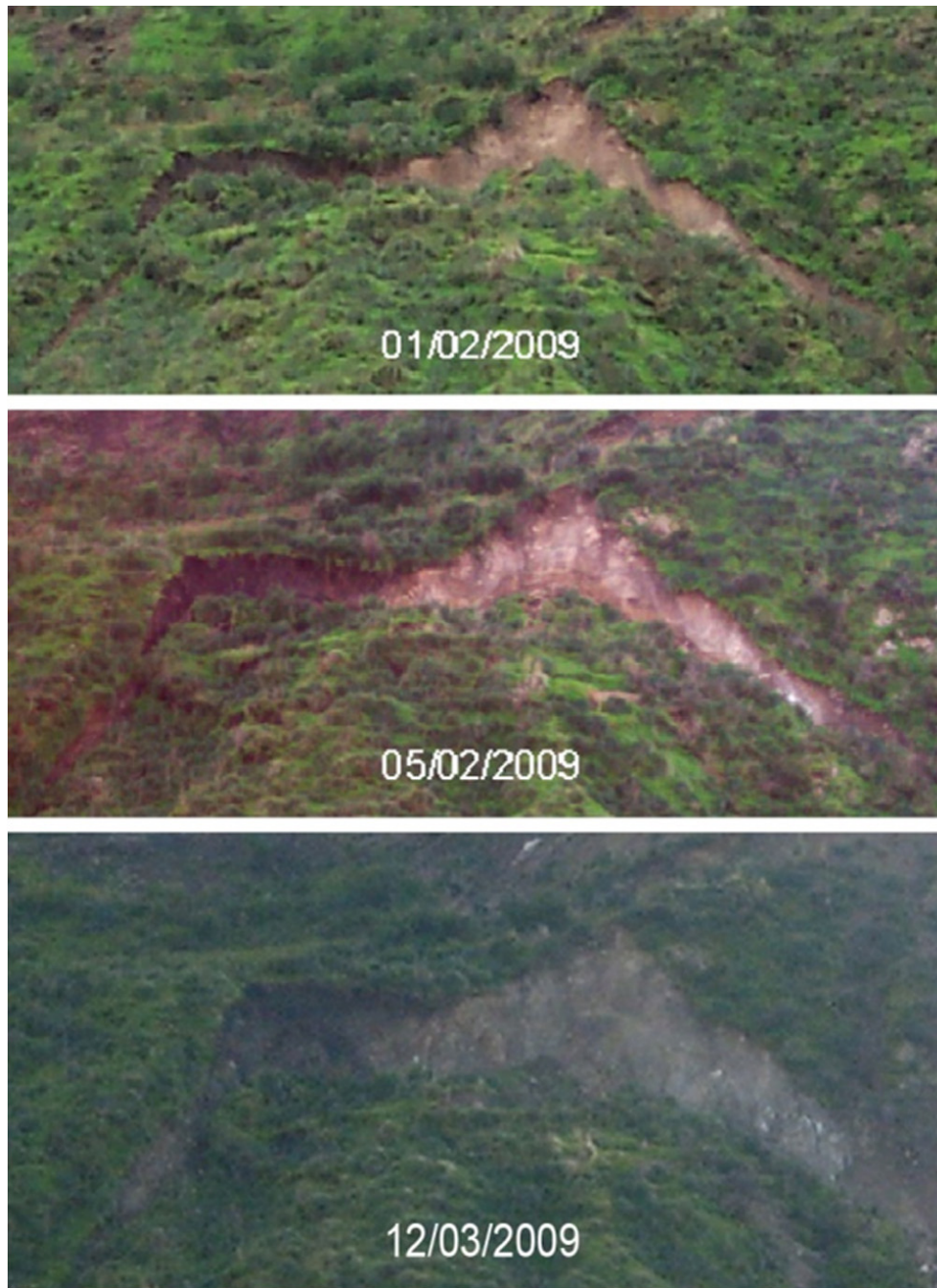
Fig. 3. Pictures of a fracture placed above the landslide. The widening of the fracture with time is clearly visible.
