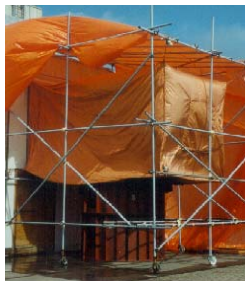
Figure 4: The VIRC as built for in-situ testing
