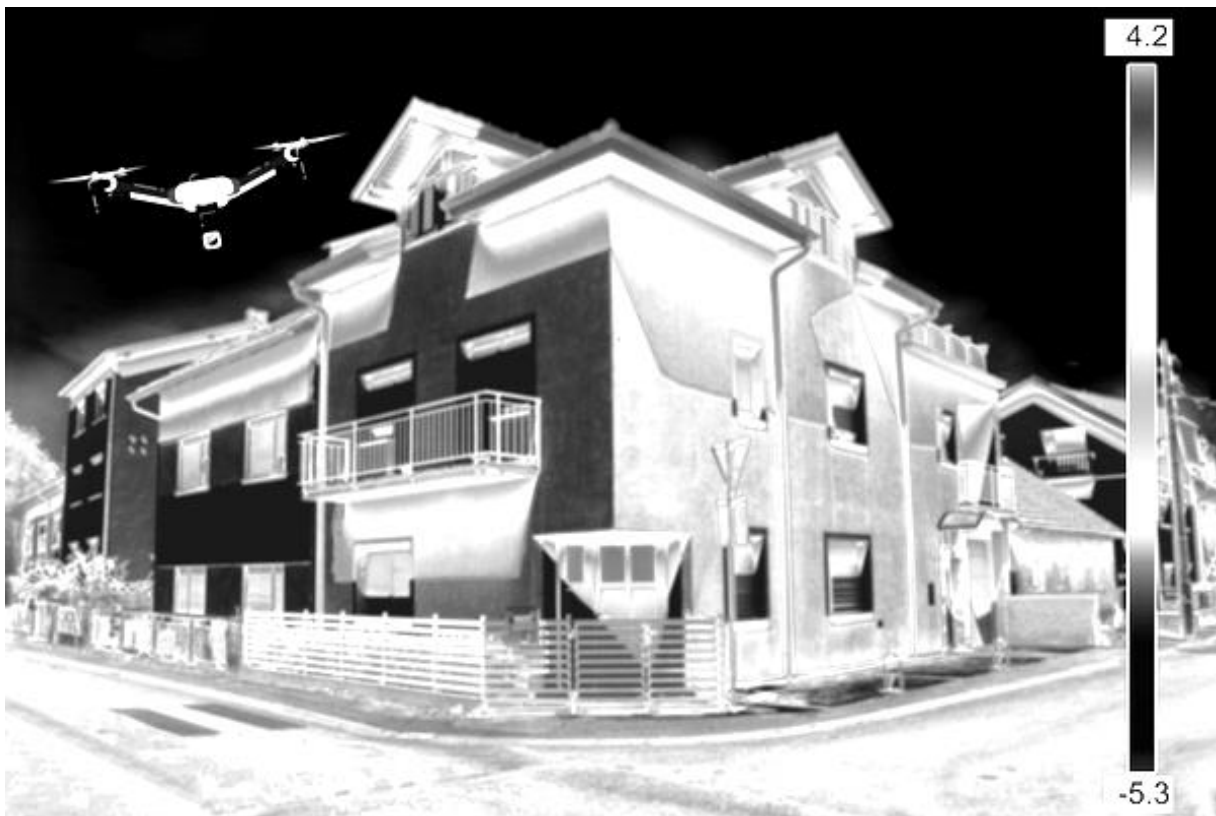
Figure 7: Example of drone thermal imaging; source [20]
