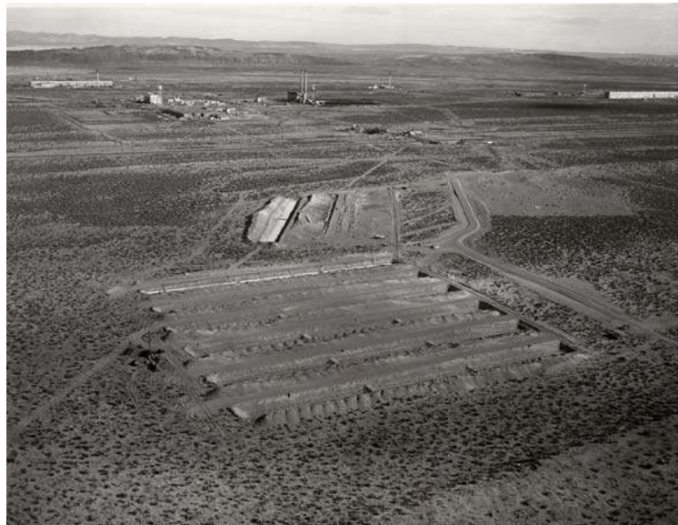
Figure 2.7. Aerial Photograph of BC Trenches Shortly After Excavation
