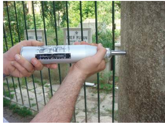
FIGURE 4: Schmidt hammer testing.
