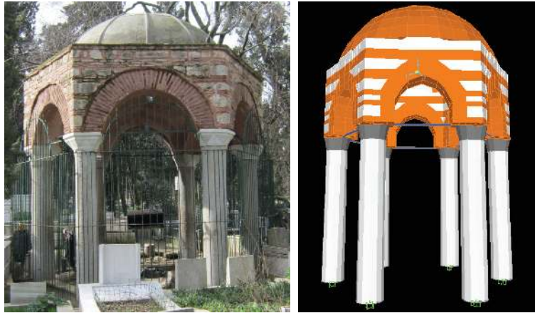
FIGURE 3: Nişancı Hamza Paşa tomb and its FEM simulation.
