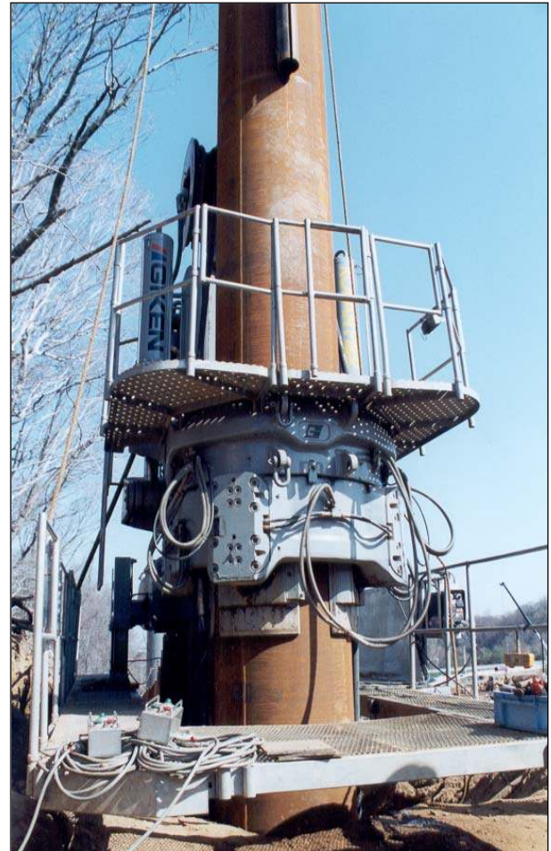
Photo 4.2. – Close up of Giken Piler with Pile
