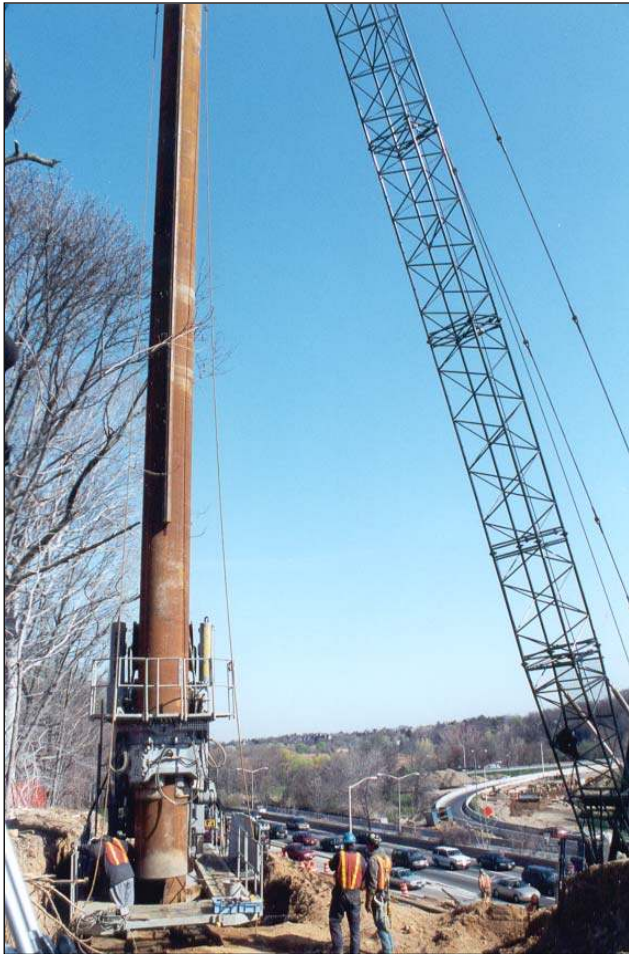
Photo 4.1. – Begin of Installation of Pile with Giken Piler
