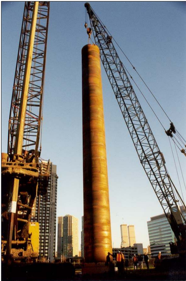
Photo 1.2. – Installation of Permanent Steel Casing
