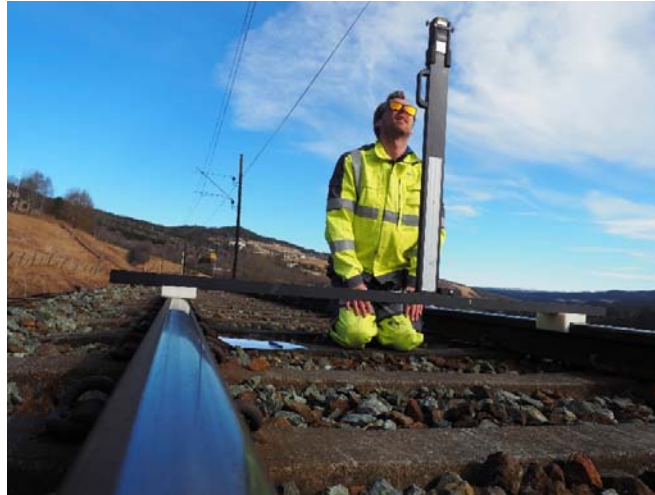
Figure 5. Measuring contact wire heights on site
