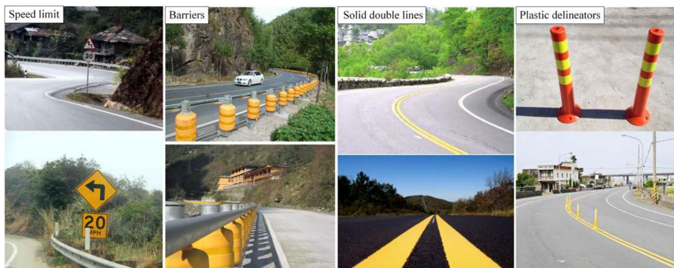
Fig. 11 Safety countermeasures for preventing passive lane departures or inhibiting the behavior of curve cutting
