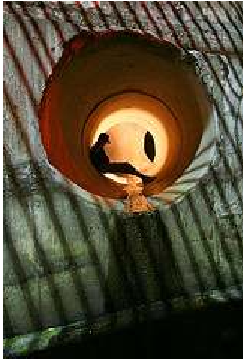
Figure 10: ‘Gatecrashed Drain’ by Mr Magoo ICU 20
