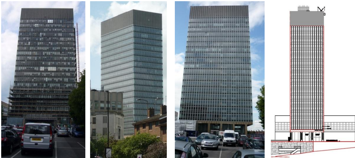
Figure 1: Views of Arts Tower: during retrofit (left), after retrofit (middle pair) and east elevation.
