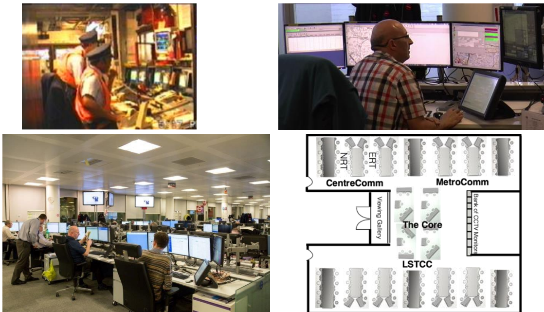
Figure 1: Examples of the domains focused on in this paper. On the top left an image of one of the control rooms considered: Piccadilly Operations room. This has one console, operated by one or two station supervisors and technologies, including various systems for monitoring traffic, making announcements, communicating with staff and operating the CCTV. On the bottom left is an image of a one area of a newer ‘multi-centre control room - the London Surface Transport and Traffic Operations Centre: LSTTOC). This is taken of part of the CentreComm area. The graphical plan (bottom right) gives a sense of the overall space where over 100 staff are located working for three principal operations organizations (CentreComm, MetroComm and LSTCC). These are located in different zones. Top right is an image focusing on one ‘work station’ within Centrecomm.
