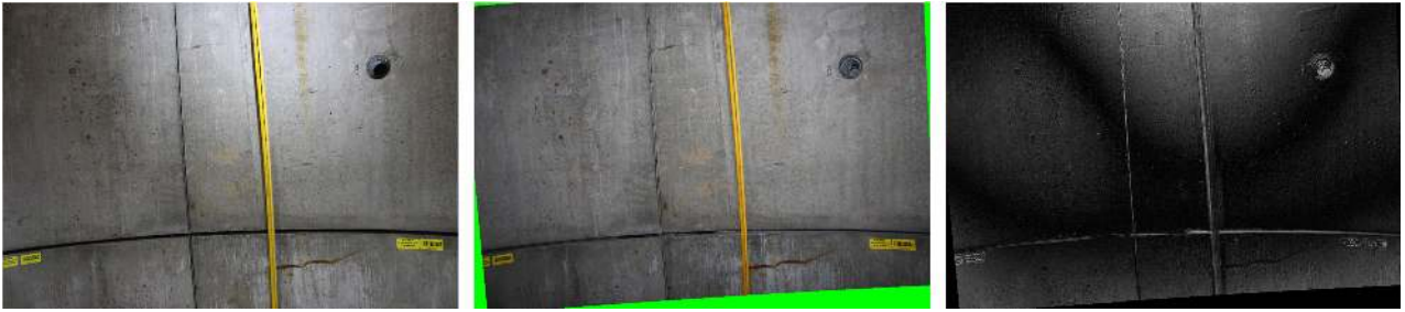
Fig. 2 Sources of nuisance variability. From left to right: new query image with no relevant change; warped matching image from database; absolute difference image, with brighter areas indicating larger changes. All differences observed in this final image are caused by nuisance variability rather than relevant change. Such nuisances include low frequency contrast changes across the tunnel lining, hard shadows around off-lining geometry and glare from specular surfaces. They are caused here by the changes in camera position and lighting.
